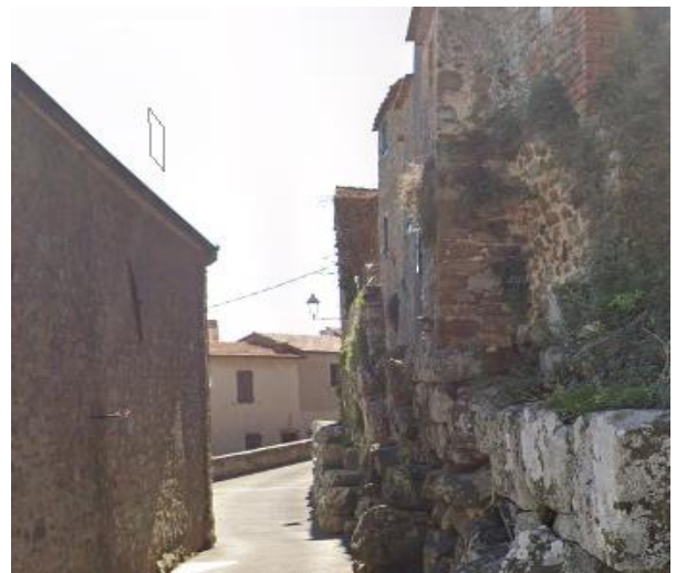
26 last stretch Cyclopean walls
