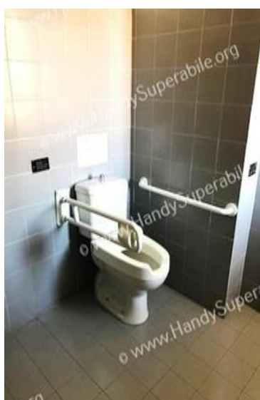
38 toilets and grab bars
